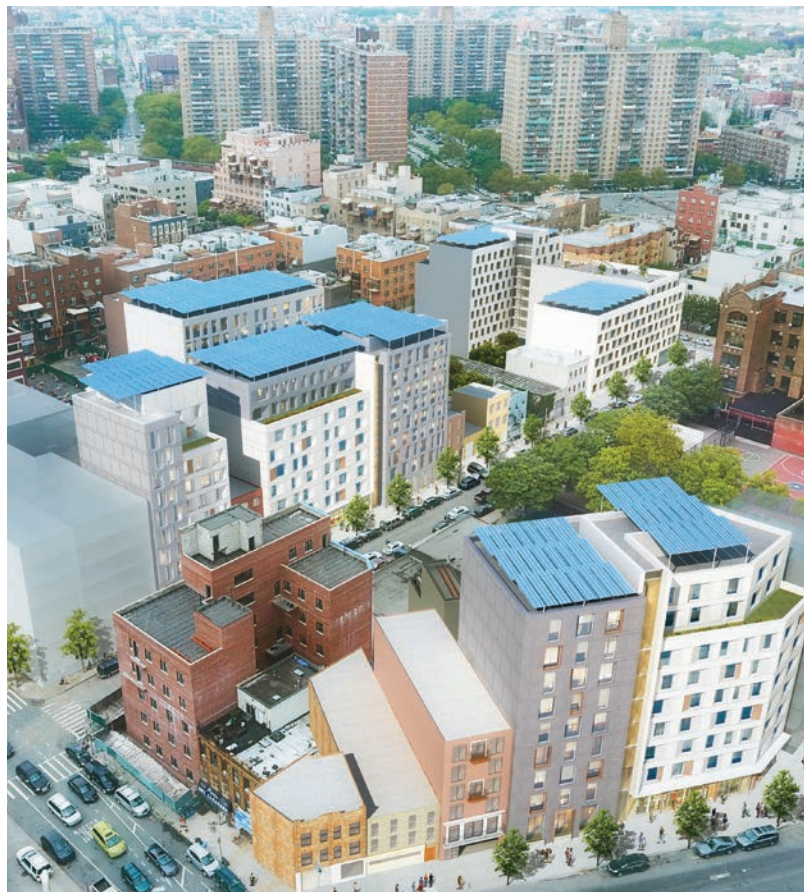
United Neighborhood Partners: Coming Together to Build Affordable Housing in the Broadway Triangle
